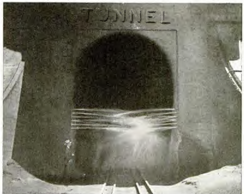
Water jets wash dirt from cars as they leave the Moffat Tunnel
